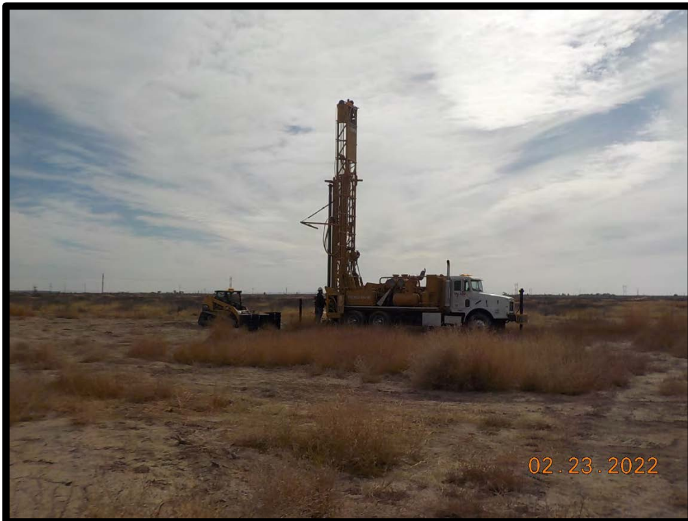
PHOTOGRAPH NO. 4 – A view of the air rotary soil boring activities at the “SB-2” location on February 23, 2022. The view is towards the southwest . (Approximate GPS: 32.724355, -104.346186)
