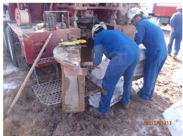
Placing the bentonite seal, MW-2 3/13/15
