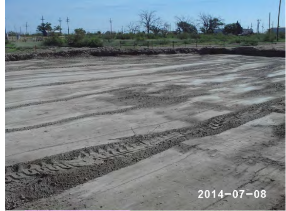
Padding above the liner, facing northeast 7/8/2014
