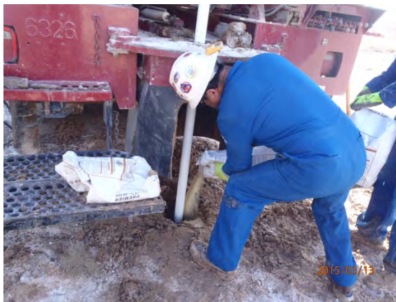
Adding the sand pack, MW-2 3/13/15
