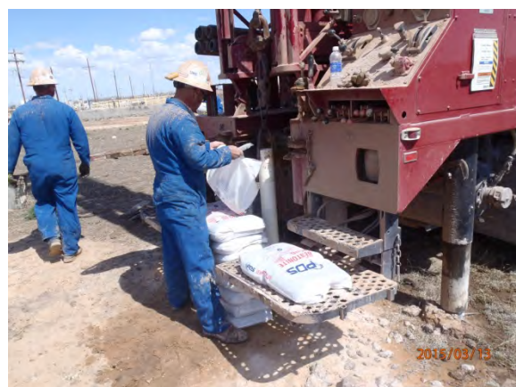
Placing the bentonite seal, MW-1 3/13/15
