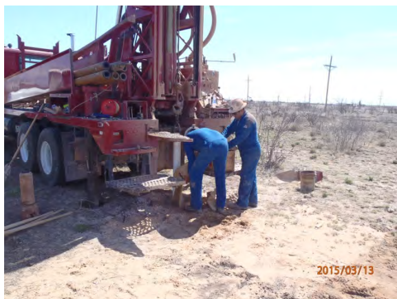
Adding the sand pack, MW-1 3/13/15
