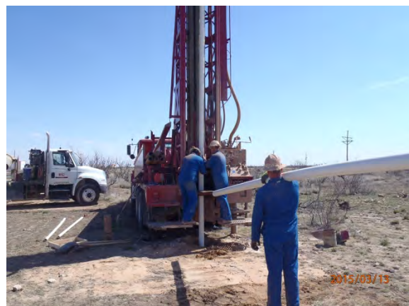
Installing casing in MW-1, facing east 3/13/15
