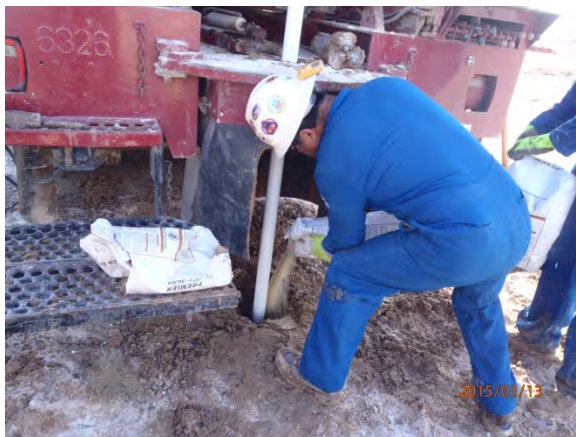
Adding the sand pack, MW-2 3/13/15
