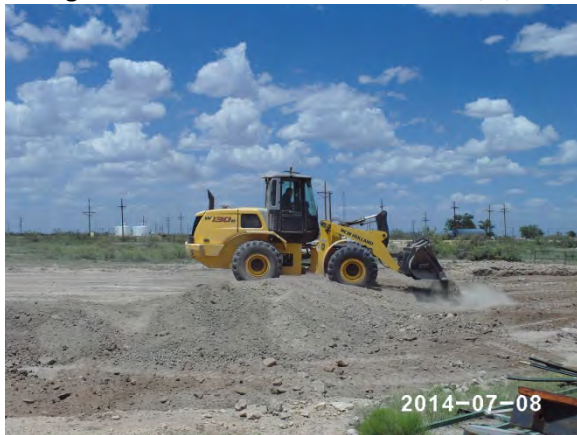
Backfilling the excavation, facing north 7/8/2014
