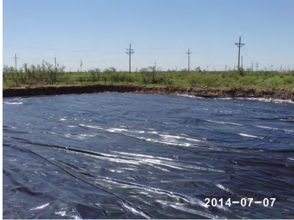
20-mil poly liner installed at 3 ft bgs, facing southeast 7/7/2014
