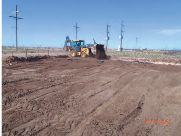
Backfilling above the liner, facing southwest 3/27/2015
