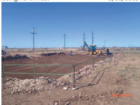
6" padding of topsoil, facing southwest
