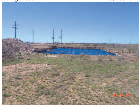
20-mil poly liner installed at 2.5 ft bgs, facing west
