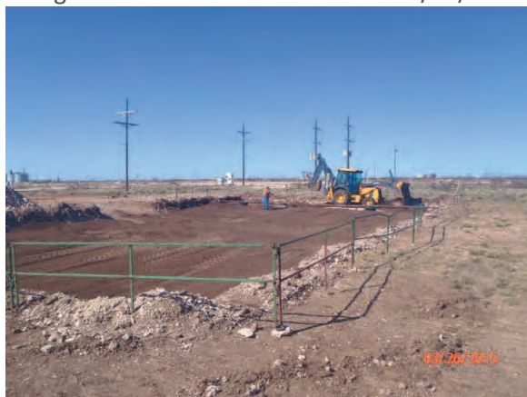
6" padding of topsoil, facing southwest 3/26/2015
