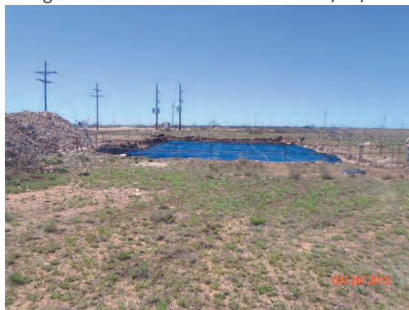
20-mil poly liner installed at 2.5 ft bgs, facing west 3/26/2015
