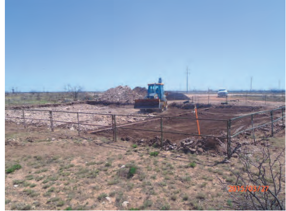
Backfilling the site with caliche rock, facing southeast 3/27/2015
