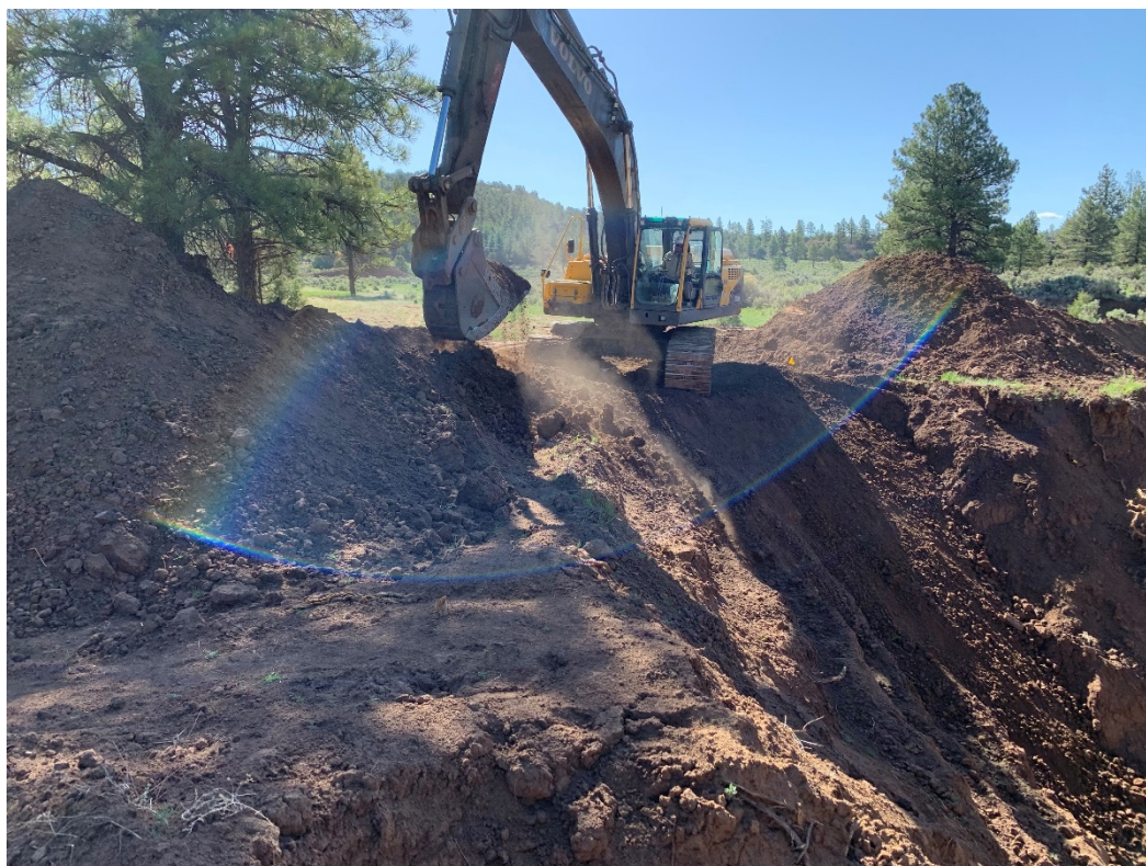
Photo 3: Pipeline excavation, March 11, 2021.
