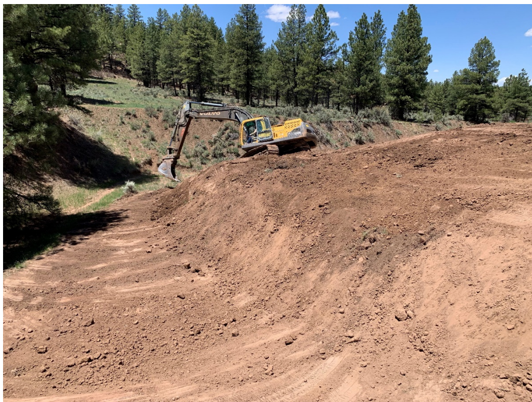
Photo 4: Excavation backfilling, May 2021.
