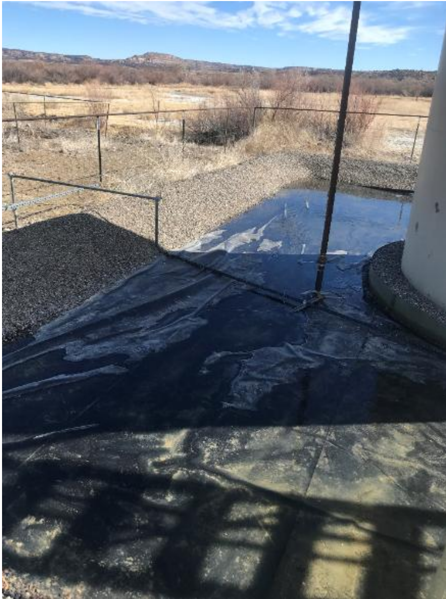
Liner integrity demonstration – after snow melt 2/4/2021
