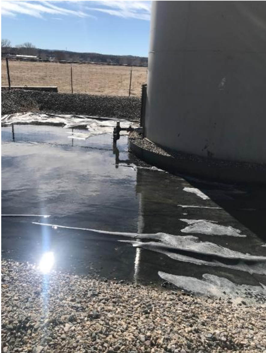
Liner integrity demonstration – after snow melt 2/4/2021
