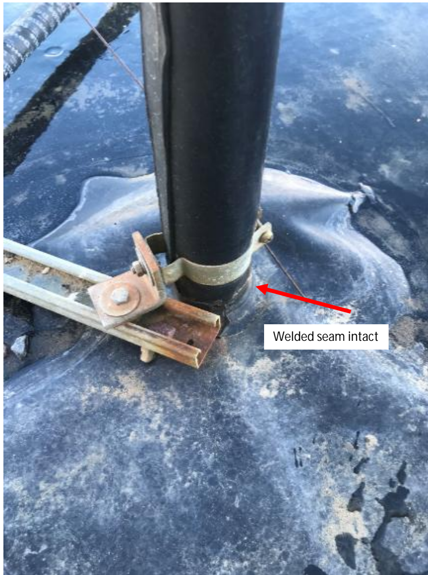
Liner integrity demonstration – after snow melt 2/4/2021
