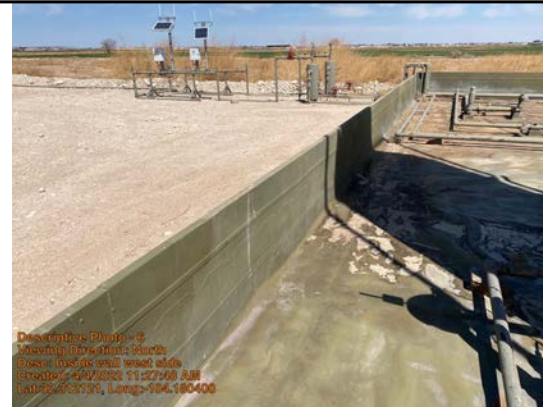
Inside wall west side
