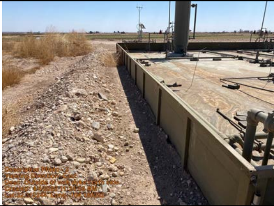
Outside of wall dyke north side.
