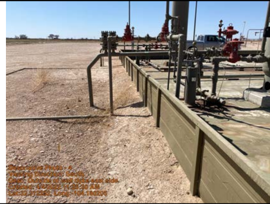
Outside of wall dyke east side.
