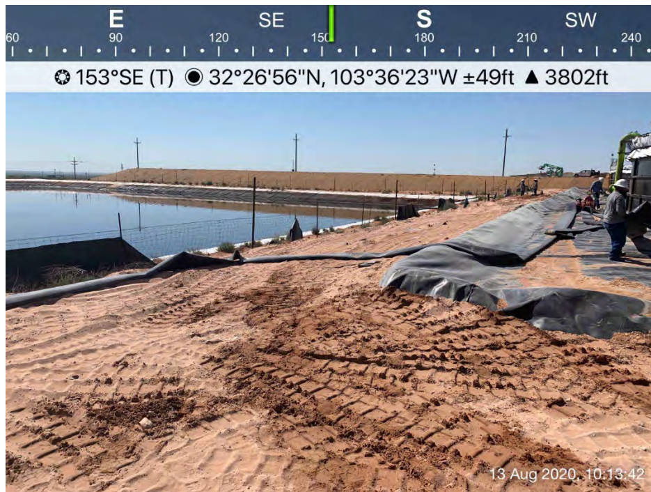
High pressure lay flat lines within spill area viewing southeast
