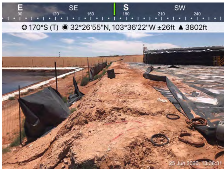
Spill on earthen embankment and liner viewing south
