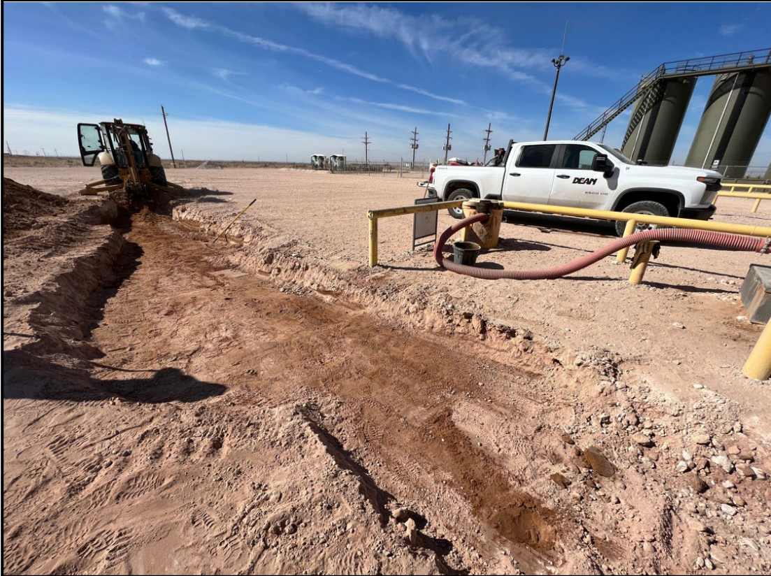
Direction: South view, note pad breakthrough to topsoil layer underneath facility, 03/03/2022.
