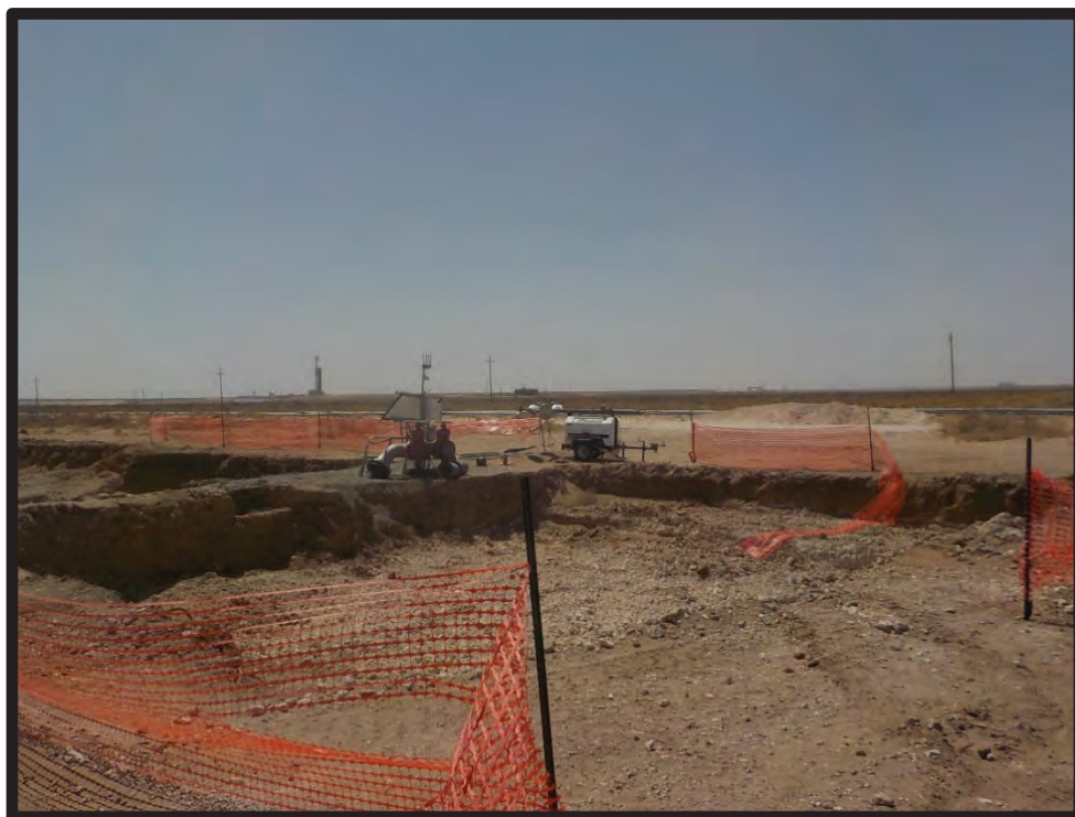
PHOTOGRAPH NO. 1 – A view of the northern excavation/remediation area at the Site during the March 29, 2022 confirmation sampling activities. The view is towards the southwest.
