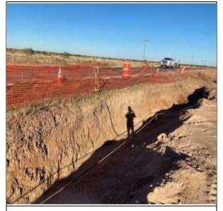
Photograph No.4 Description: Excavation of spill path on right-of-wayexposed utility lines
