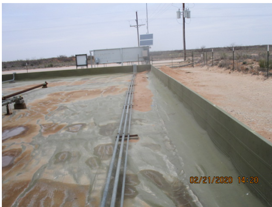
View of sediment and minor pooling within lined secondary containment
