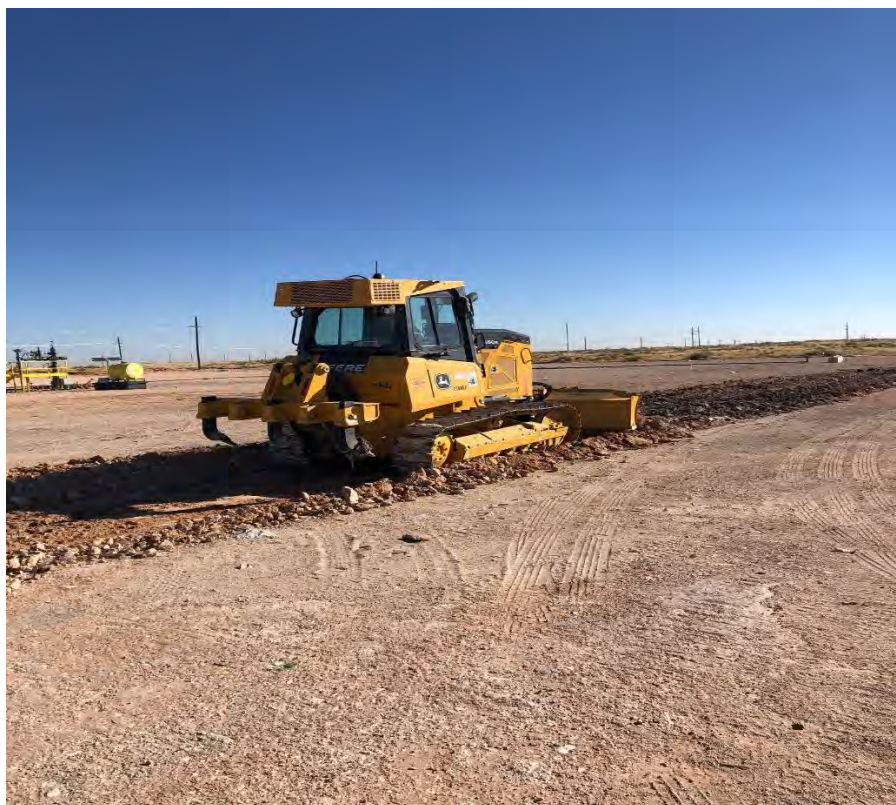
Photo 1. View of bulldozer scraping impacted soil in the area of excavation
