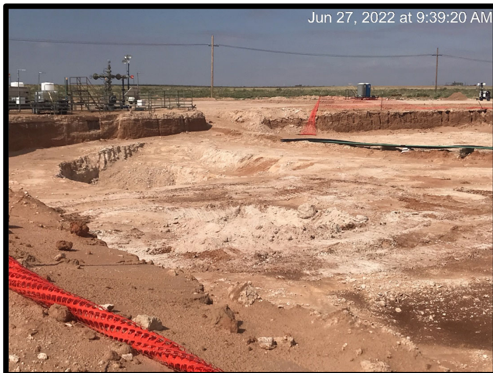
PHOTOGRAPH NO. 3 – A view of the Site upon completion of over-excavation activities in the “B-80” sample area on June 27, 2022.
