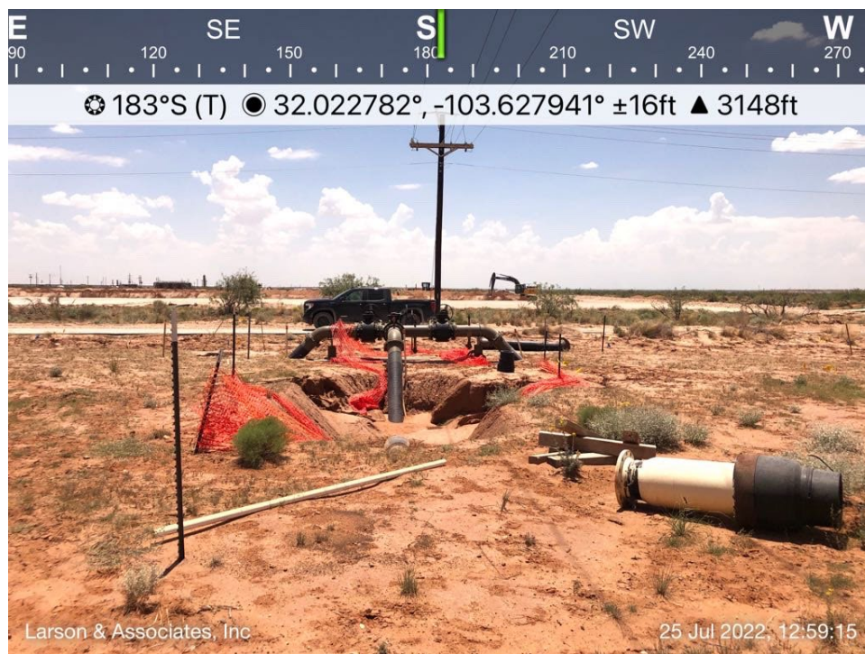
Release source and impacted area viewing south
