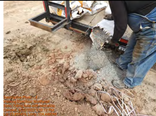
Filling hole with bentonite
