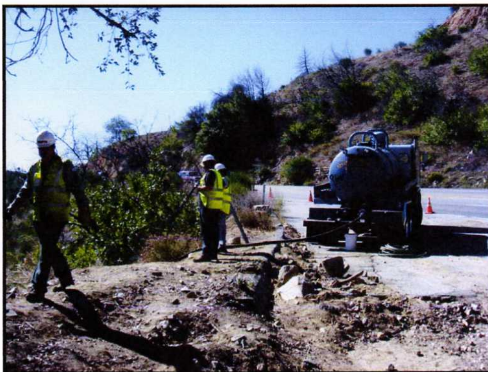
Photo 16: October 20, 2006 Remedial action at Highway 18 spill site - HMHTTC Vacuum Truck with Liquid Remediate™ at top of Ravine.
