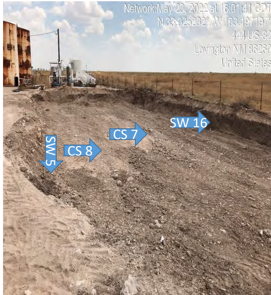
View Southwest – Sample locations Confirmation Sample 7 (5'EB), Confirmation Sample 8 (5'EB), Side Wall 16, and Side Wall 5 (flagged). Blue arrows identify pin flags.
