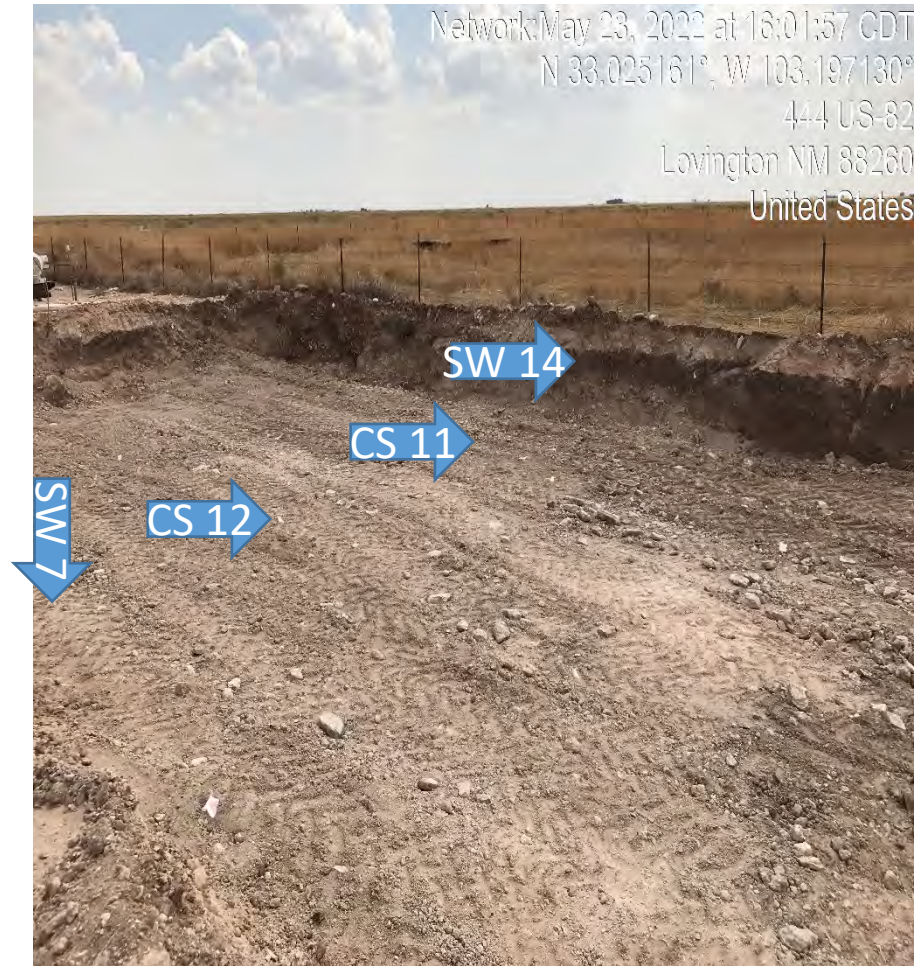
View Southwest – Sample locations Confirmation Sample 11 (5' EB), Confirmation Sample 12 (5' EB), Side Wall 14, and Side Wall 7 (flagged). Blue arrows identify pin flags.
