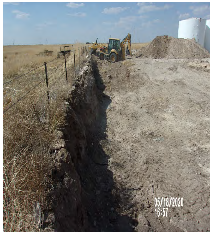
View North – Remediation activities (excavating impacted material to a depth of 5 ft bgs.) ongoing.
