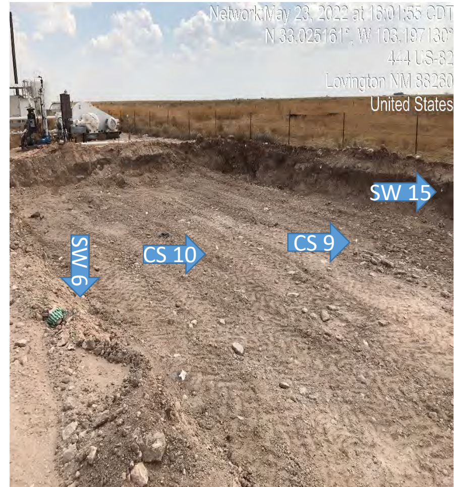
View Southwest – Sample locations Confirmation Sample 9 (5'EB), Confirmation Sample 10 (5'EB), and Side Wall 15, and Side Wall 6 (flagged). Blue arrows identify pin flags.
