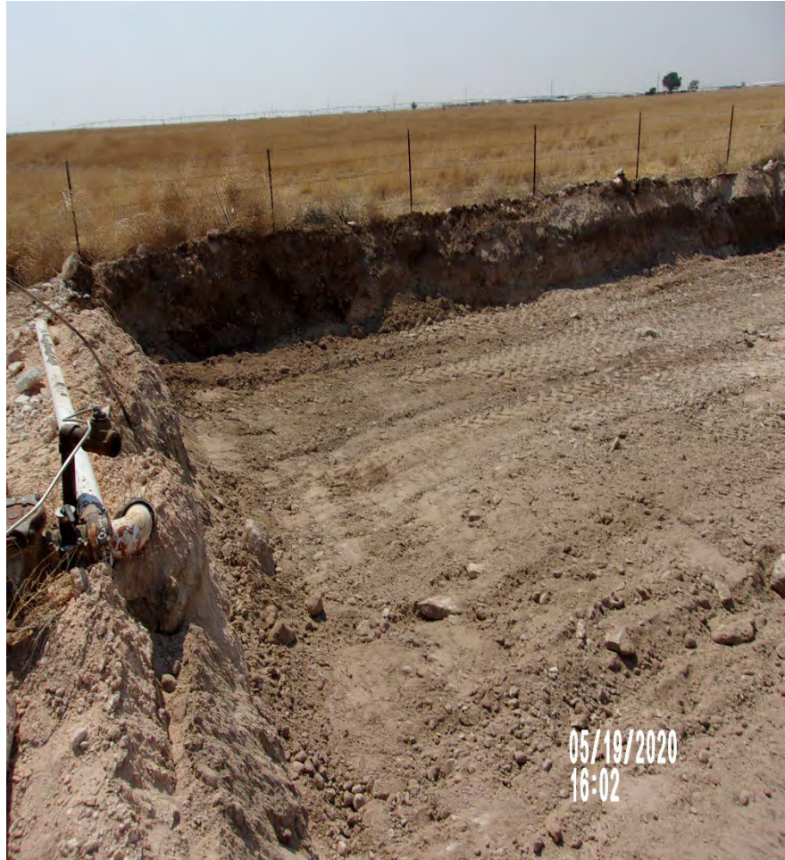
View Northwest – Remediation activities (excavation of impacted material to a depth of 5 ft bgs.) completed.
