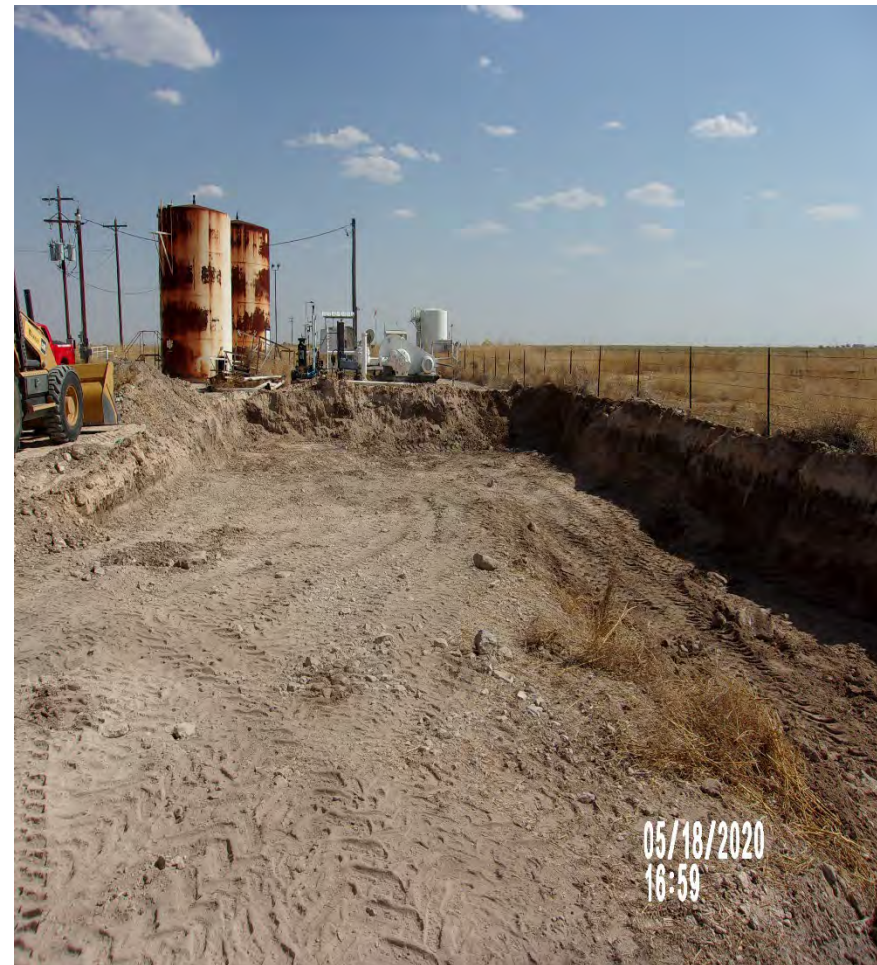
View South – Remediation activities (excavating impacted material to a depth of 5 ft bgs.) on-going.
