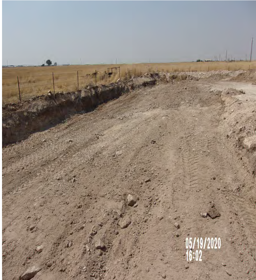
View North – Remediation activities (excavation of impacted material to a depth of 5 ft bgs.) completed.
