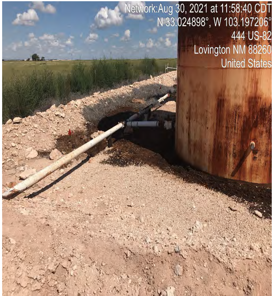
View North – Origin of spill. Cause of the release due to corrosion of piping. Note a portion of the spill flow path (dark brown staining) within the release footprint.
