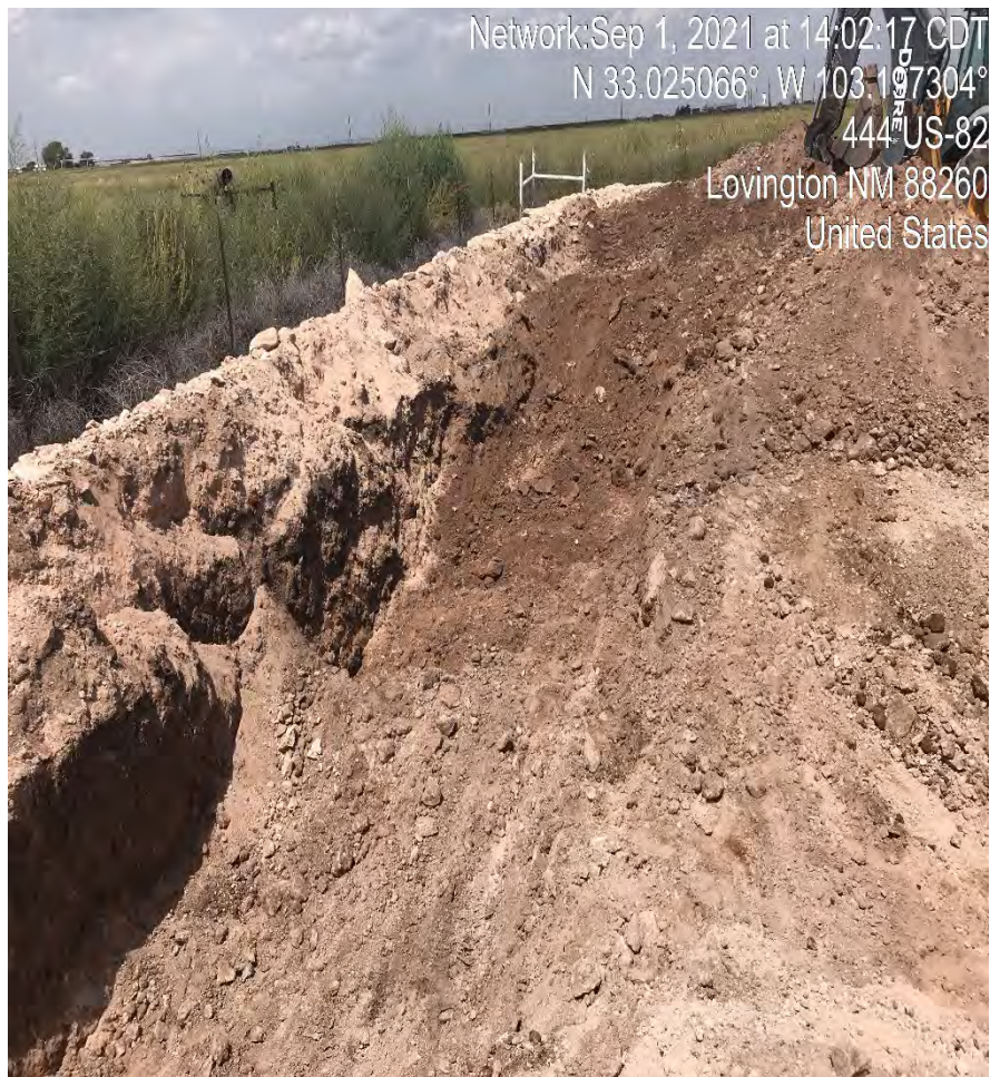
View North – Excavation activities were conducted by a third-party contractor.
