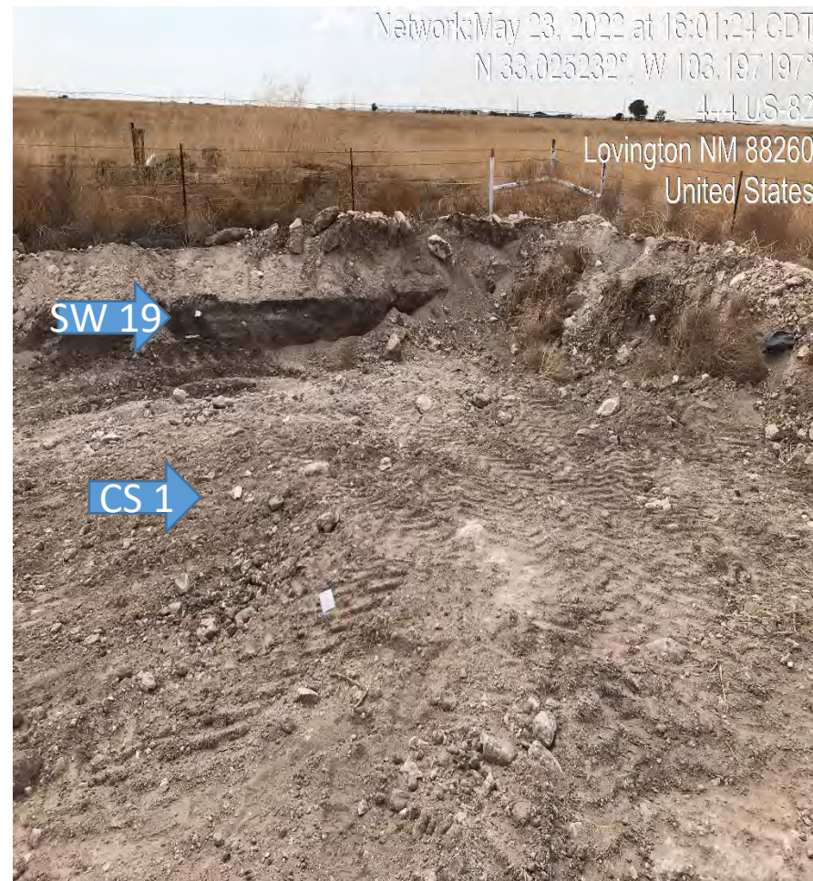
View Northwest – Sample locations Confirmation Sample 1 (5'EB) and Side Wall 19 (flagged). Blue arrows identify pin flags.
