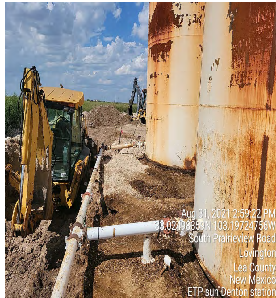
View North – Excavation activities by a third-party contractor ongoing.
