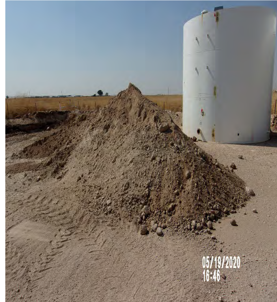
View South – Excavated impacted stockpiled material to be exported offsite to an approved disposal facility.
