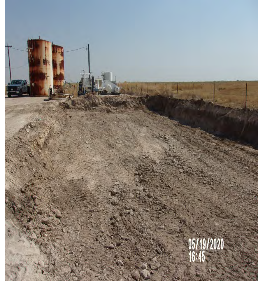
View South – Remediation activities (excavation of impacted material to a depth of 5 ft bgs.) completed.
