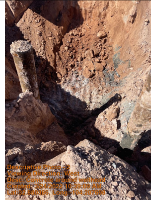
Concrete around wellhead
