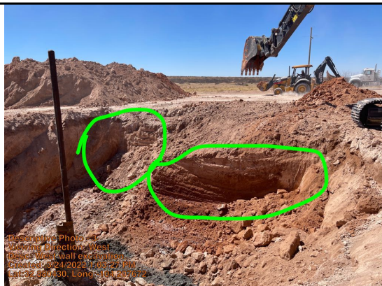
West wall excavation. All of wall excavated to visibility and odor clearance
