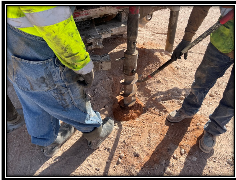
Picture 7: Soil Boring Drilling Activities
