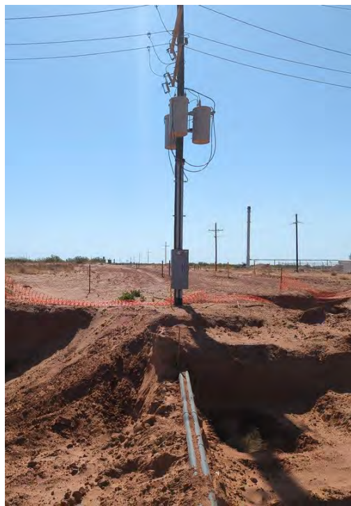
Figure 3: The utility pole within the east defer area. The buried powerline extends from the utility pole and transects west toward the production facility. Photograph is viewing east.
