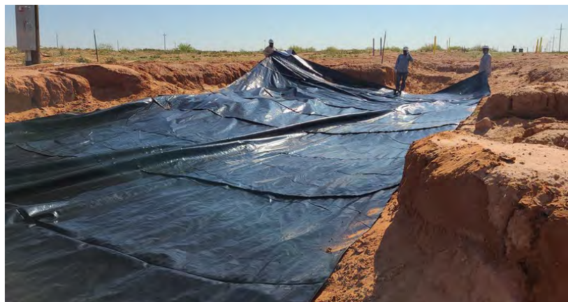
Figure 1: Lining the eastern portion of the remediation area. Photograph is viewing east-northeast as captured from grid G-12.
