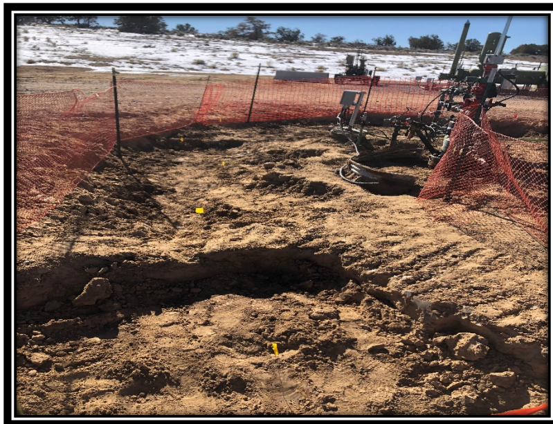
Picture 4: South Excavation with Sampling Points
