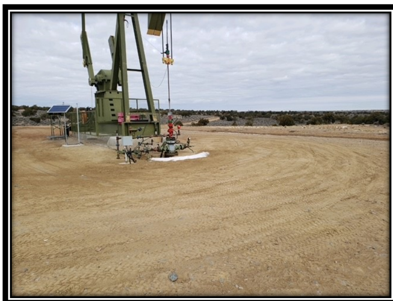
Picture 6: Backfilled and Recontoured Area
