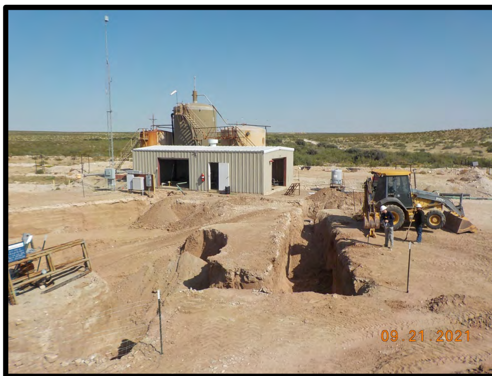
PHOTOGRAPH NO. 4 – A view of the trenching activities completed for the new injection line to the wellhead. The view is towards the north.
