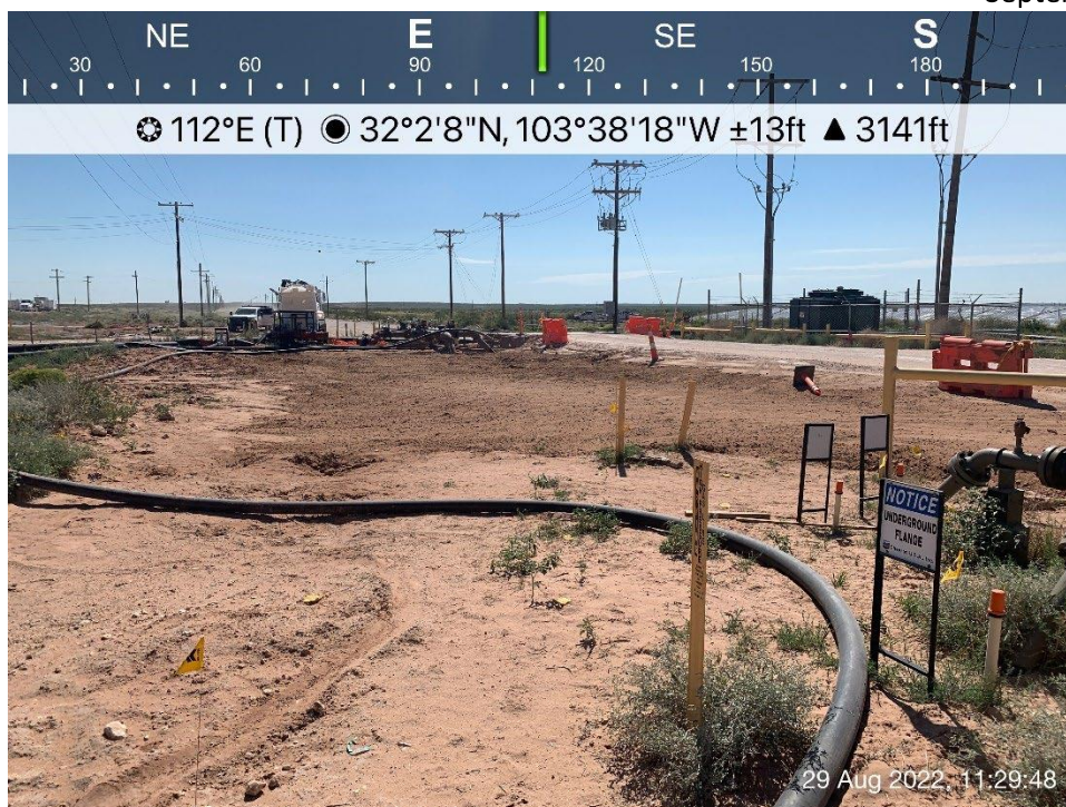
Seeded backfilled area viewing east, August 29, 2022
