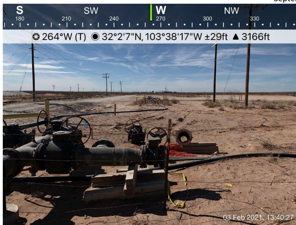
Impacted area (nAPP2036347592) viewing West, February 3, 2021
