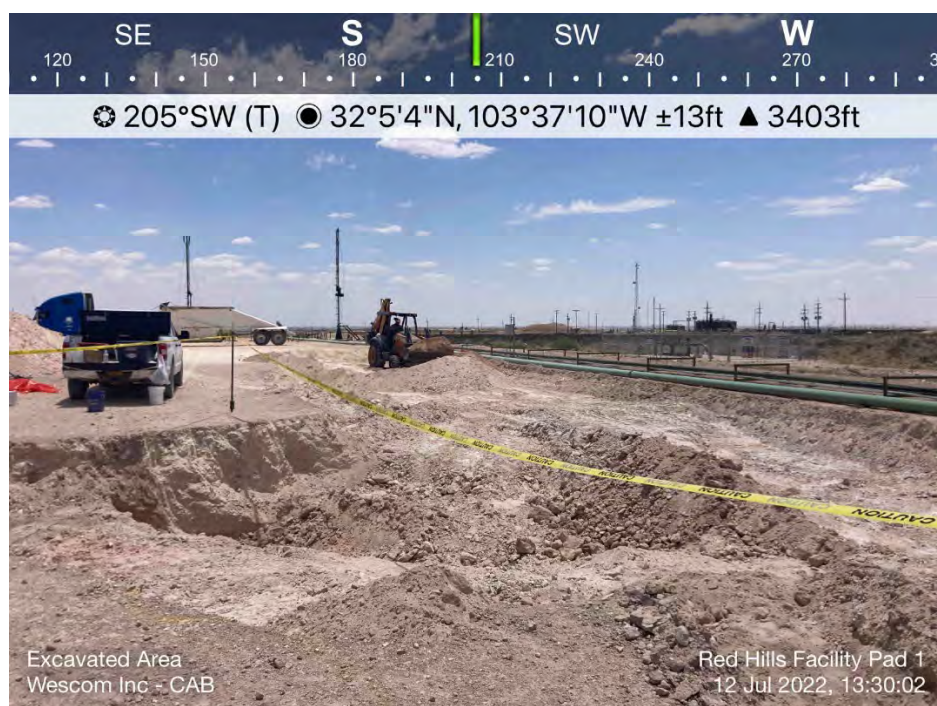
Excavated Area - On Pad Removal of Contaminated Soil
