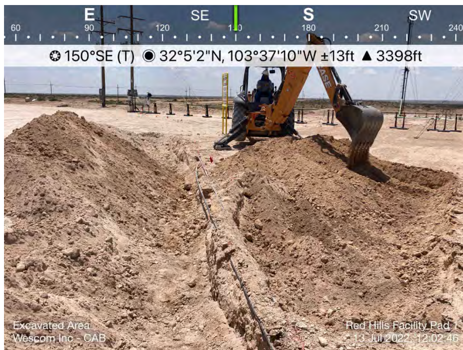
Excavation Around Electrical Line
