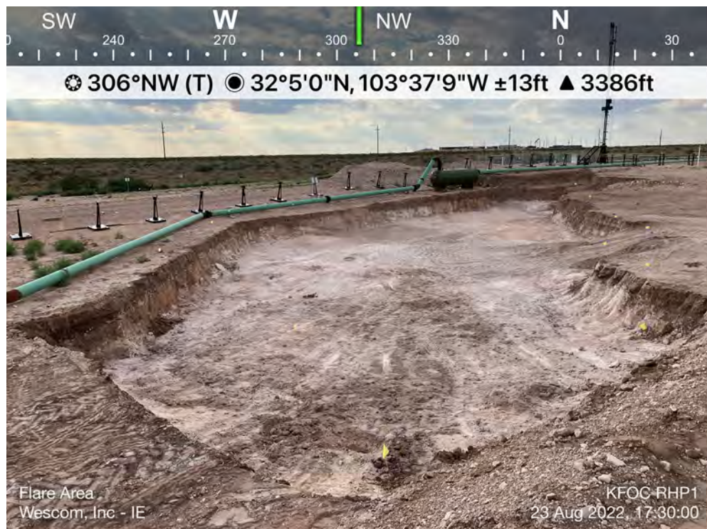
Completed Excavation - Flare Containment
