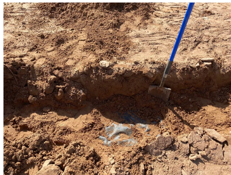
Photograph 4: Previously installed liner near SP-4 exposed.
