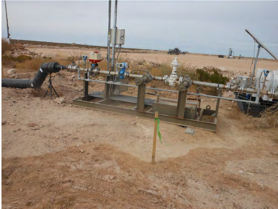
View north at meter station and camel back – point of release at poly piping
