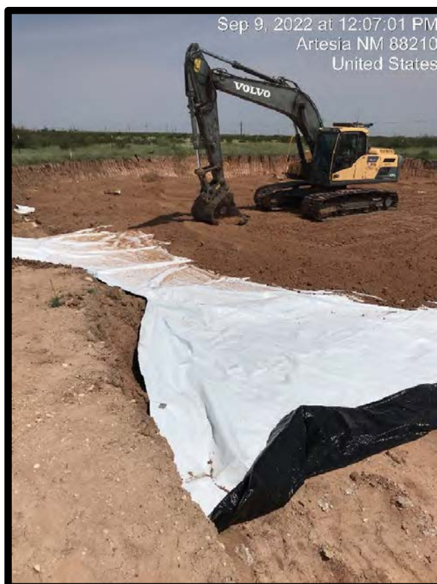
PHOTOGRAPH NO. 4 – A view of the protective over-excavation and liner installation activities. The view is towards the northeast. (Approximate GPS: 32.605240, -104.552039)
