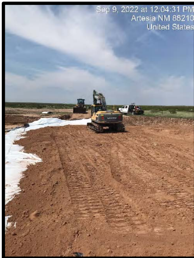
PHOTOGRAPH NO. 5 – An additional view of the protective excavation and liner installation activities. The view is to the west. (Approximate GPS: 32.605304, -104.551519)
