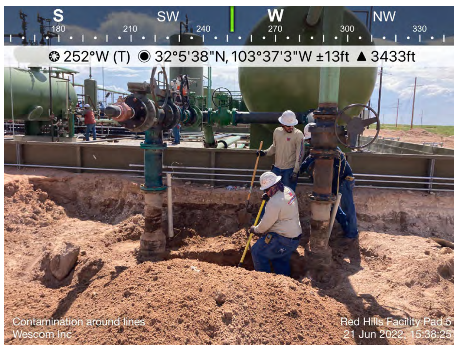
Hand Digging Around Pipelines
