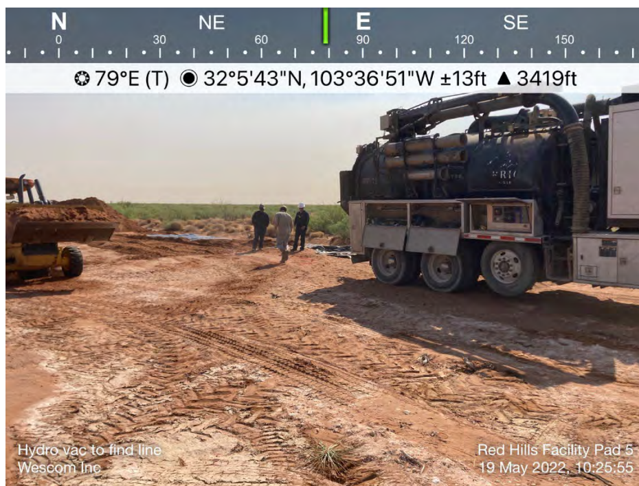
Hydrovac to Locate Pipelines
