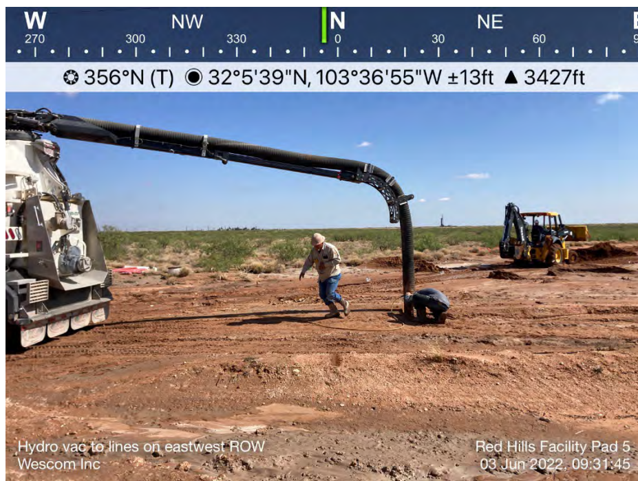
Hydrovac to Locate Pipelines on East ROW
