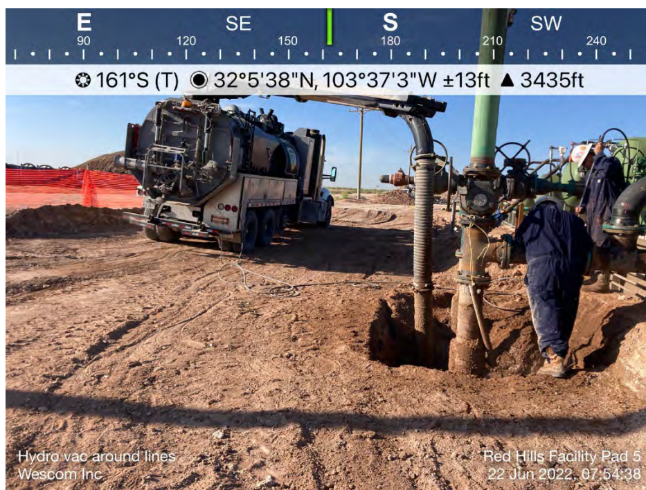
Hydrovac Around Pipelines
