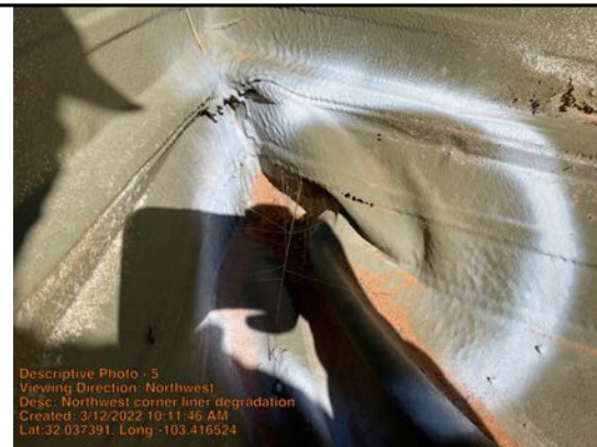
Northwest corner liner degradation
