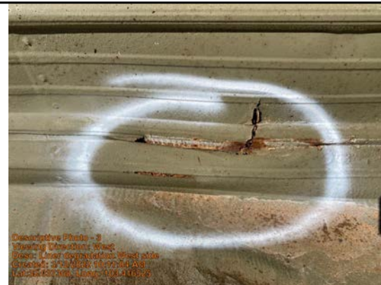
Liner degradation West side
