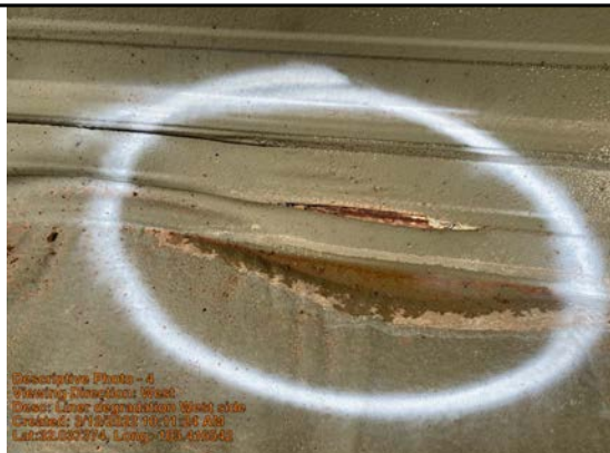
Liner degradation West side
