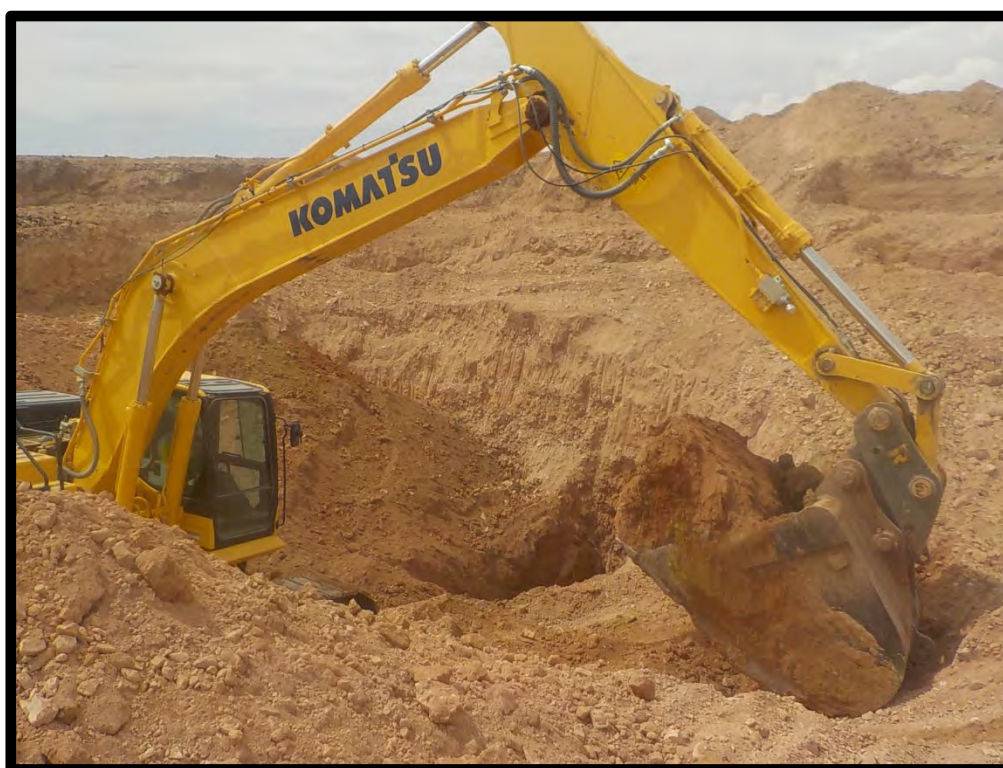
PHOTOGRAPH NO. 2 – A view of the vertical test excavation assessment process on April 27, 2022. The view is towards the southwest.
