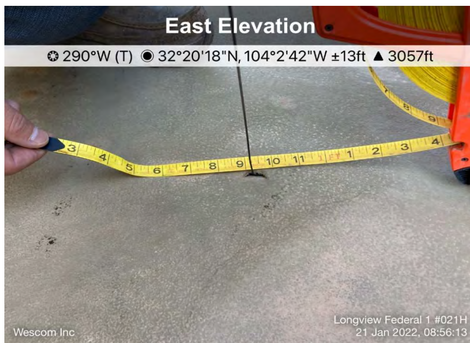
Hole at North Containment Wall (CONF05)
