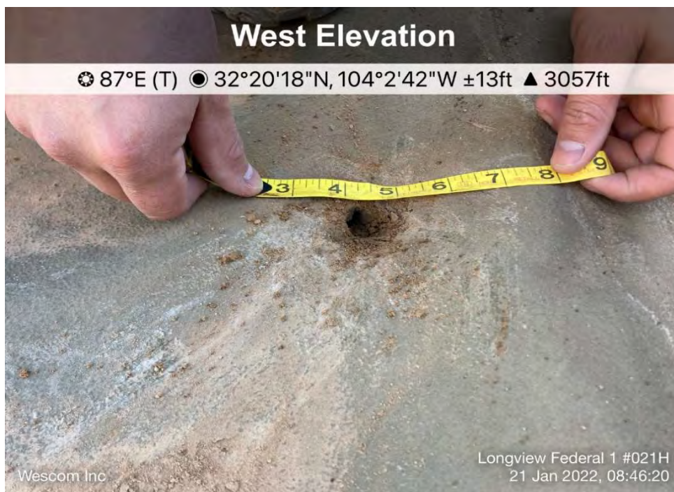
Hole at South Containment Wall (CONF07)
