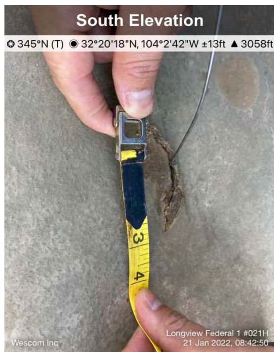
Hole on West Side of Catwalk Stairs (CONF06)
