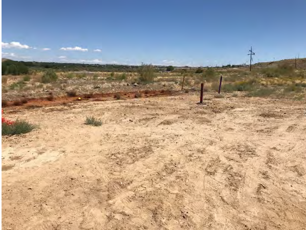
Photograph 3: MW06 completed well, 35 feet.
