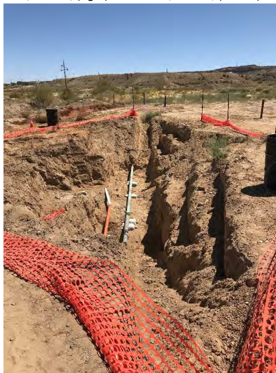
Photograph 6: Excavation looking southeast.
