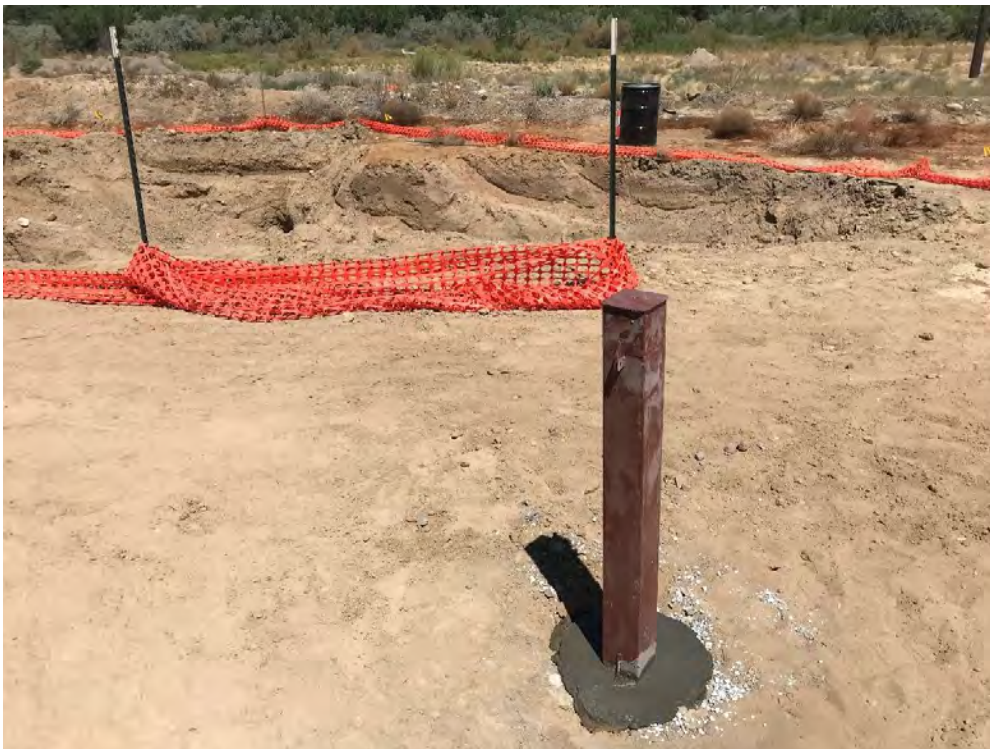
Photograph 2: MW05 completed well, 35 feet.
