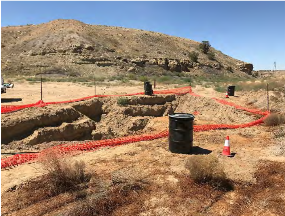
Photograph 1: Excavation looking southwest.
