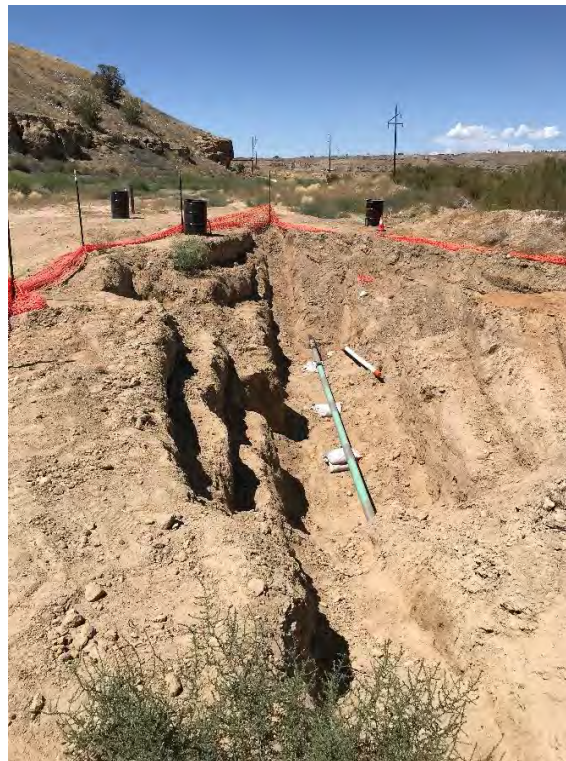
Photograph 4: Excavation looking northwest.
