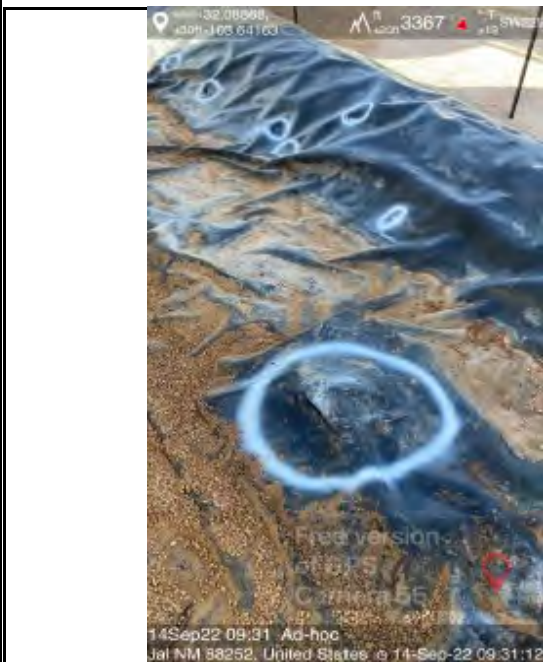
Photograph 3 Date: 09/14/2022 Description: View of tear in the liner found during remediation activities.
