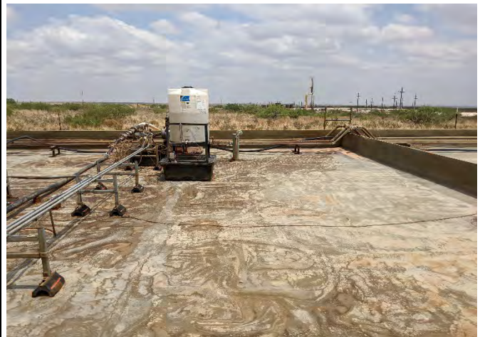
Photograph 4 Date: 6/1/2022 Description: View of the intact liner within the containment area
