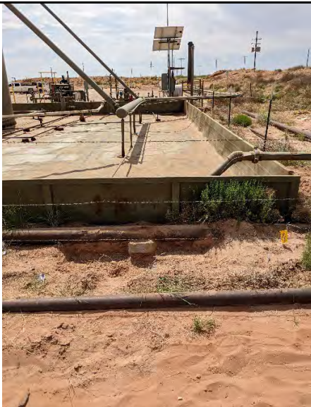
Photograph 5 Date: 6/1/2022 Description: View of the intact liner within the containment area
