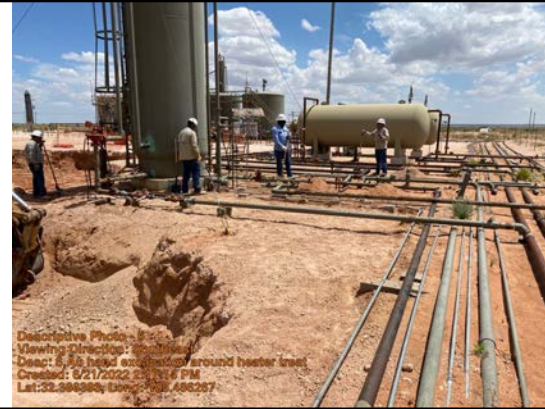
6" hand excavation around heater treater
