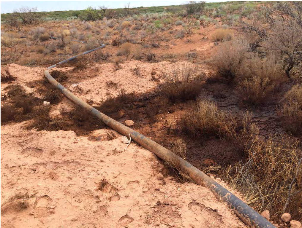
SP4 This 2019 image shows that RWO placed clean soil in certain areas of the release to absorb crude and to stabilize the release.
