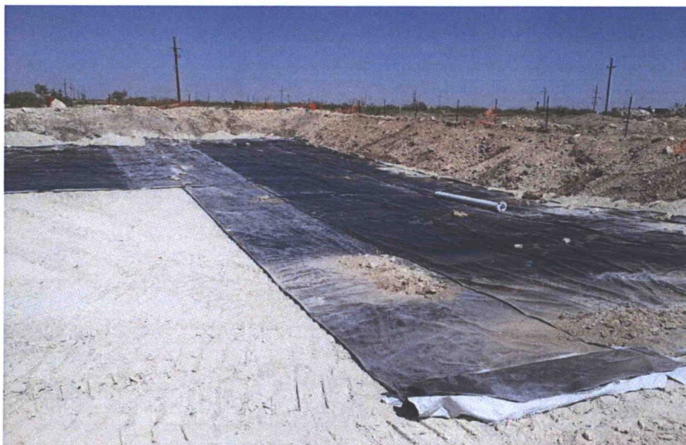
PHOTO 11: View of 20 mil poly liner installation facing northeast
