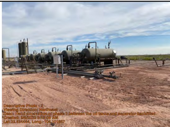
Hand excavation of phase 1 between the oil tanks and separator backfilled
