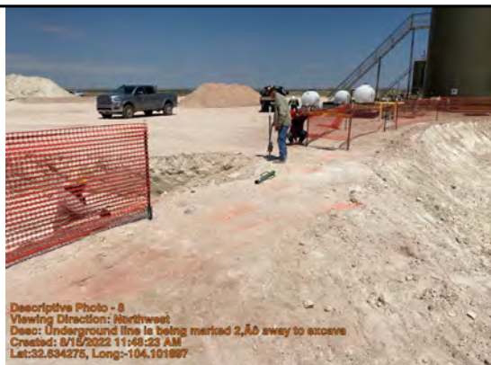
Underground line is being marked 2' away to excavate
