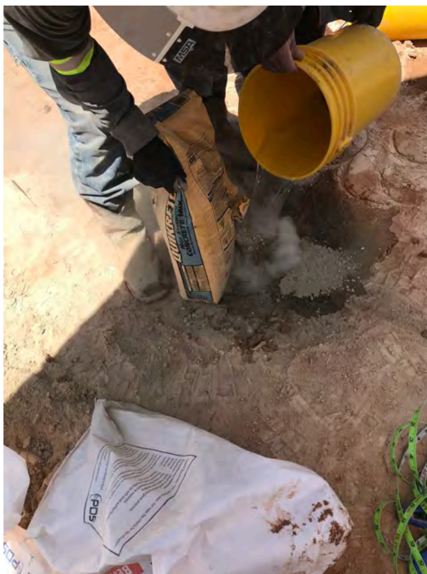
View of bentonite grout and capping soil boring at surface with concrete
