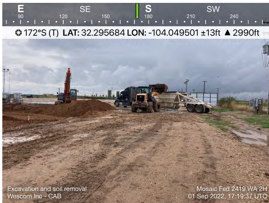
Removal of Contaminated Soil
