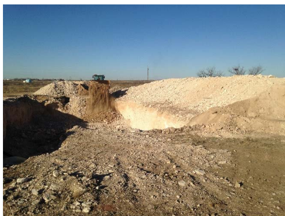
Adding clay liner and backfilling excavation, facing west
