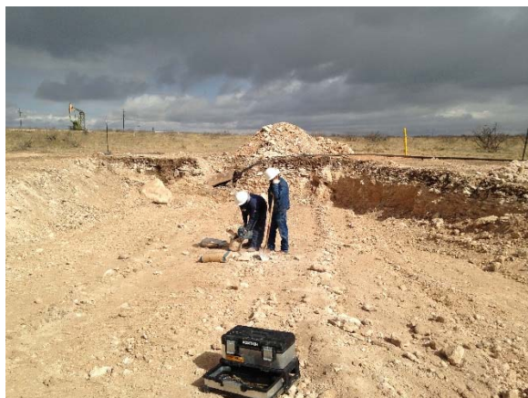
Plugging SB-1 with bentonite, facing east 2/23/2016
