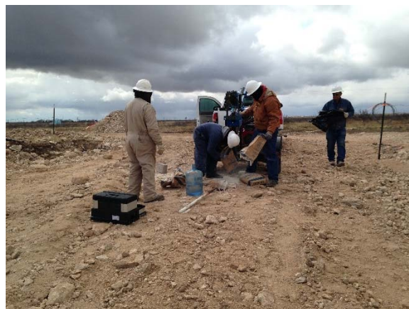
Plugging SB-2 with bentonite, facing west 2/23/2016
