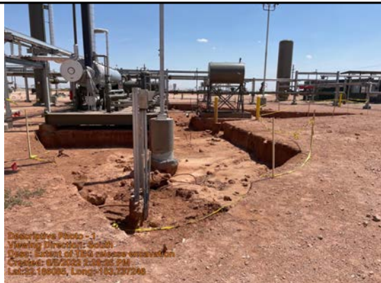
Extent of TEG release excavation
