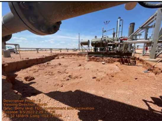
Dehy skid, TEG containment and excavation
