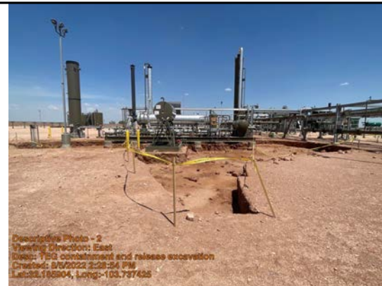
TEG containment and release excavation
