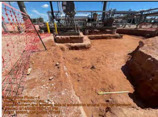
Southern and western side of excavation around TEG containment
