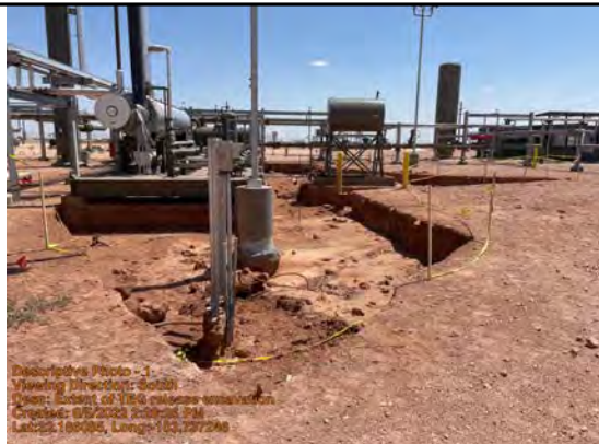
Extent of TEG release excavation
