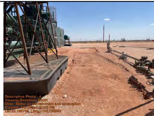
Motor oil containment and excavation
