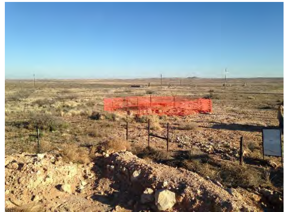
Completed 1' excavation, facing southeast 2/15/2016
