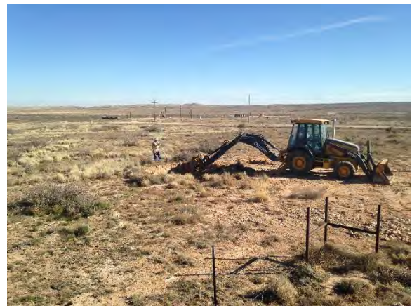
Excavating site, facing southeast 2/15/2016
