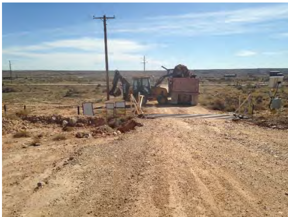
Exporting soil, facing south 2/15/2016
