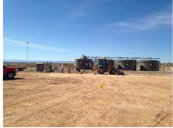
Excavating site, facing west 2/15/2016
