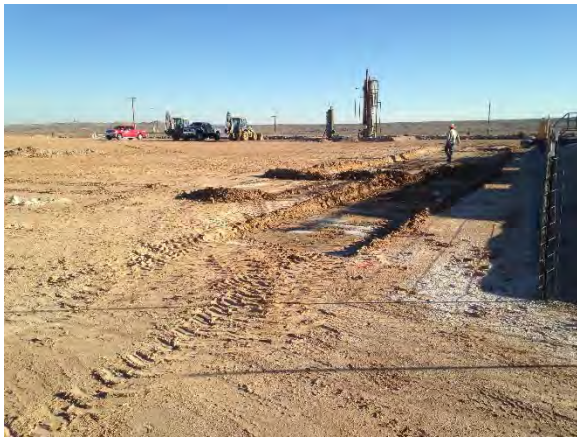
Completed 1' excavation, facing southeast 2/15/2016
