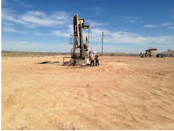
Excavating site, facing east 2/15/2016
