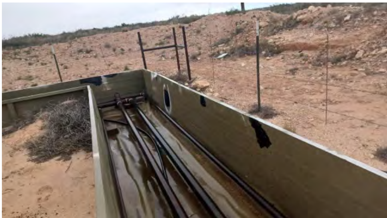
Containment Wall Repaired
