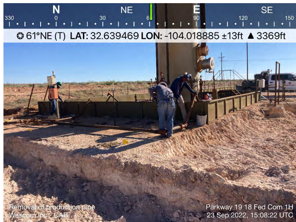
Removal of Production Pipe
