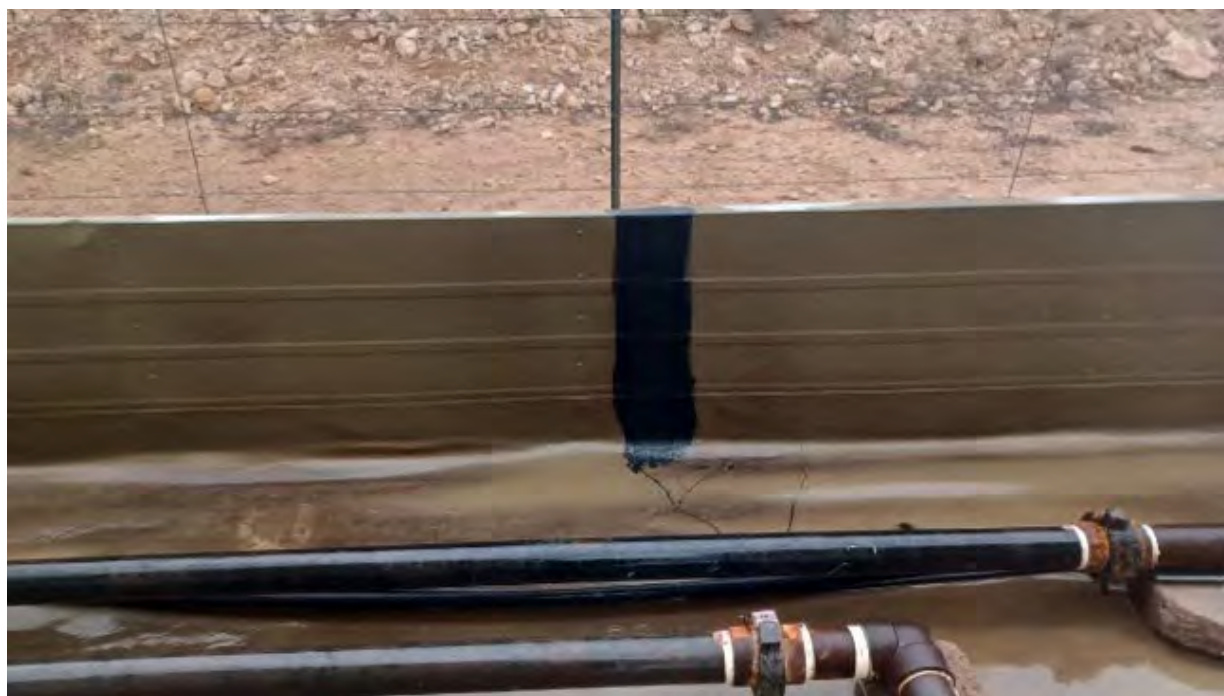
Containment Wall Repaired
