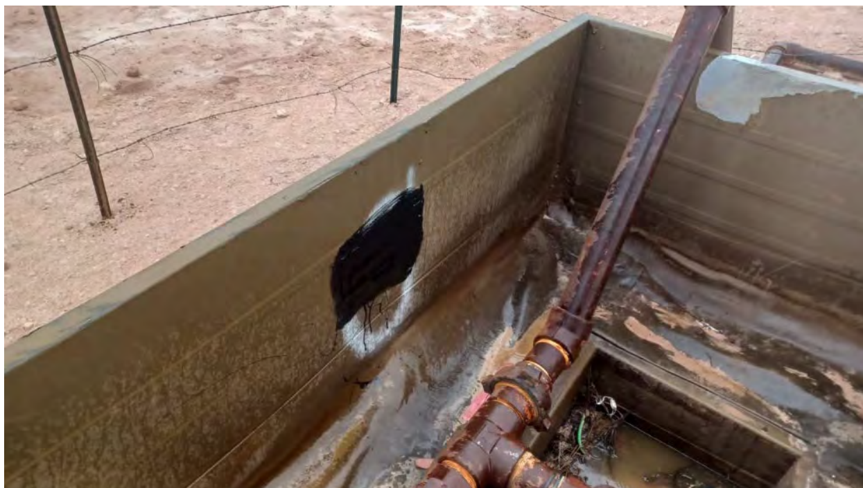
Containment Wall Repaired
