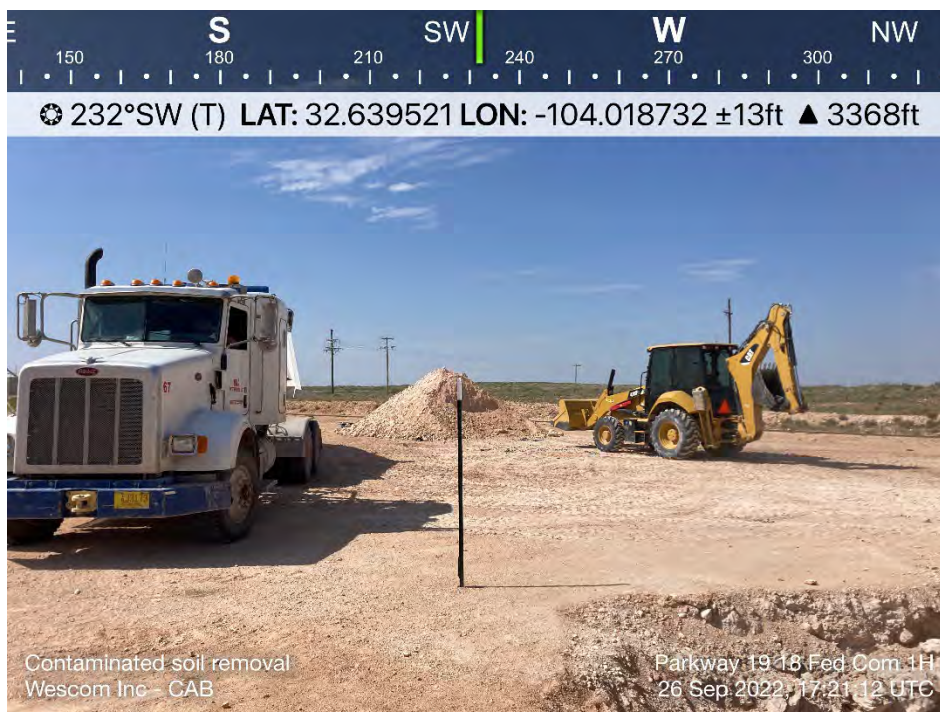
Removal of Contaminated Soil
