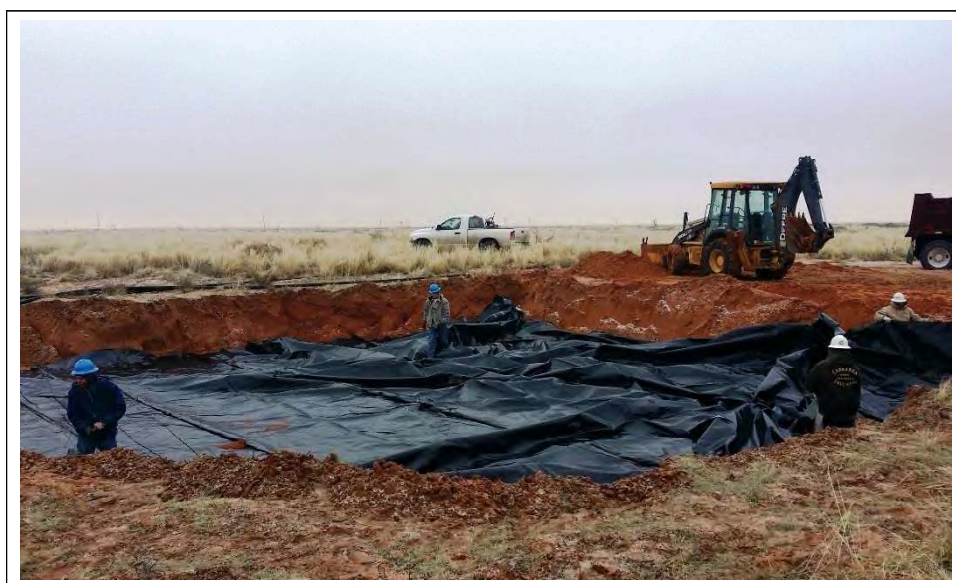
Liner Installation
