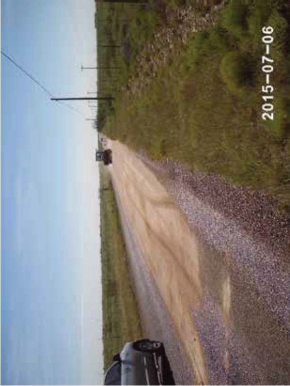
Covering spill area on road with caliche facing east
