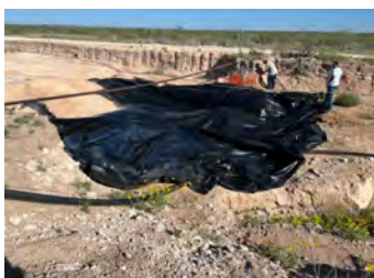
Liner installed and backfill started (9/21/22).
