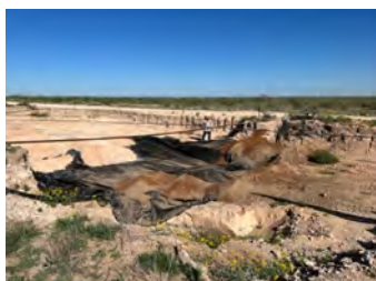
Liner installed and backfill started (9/21/22).
