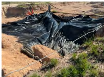
Liner installed (9/21/22).
