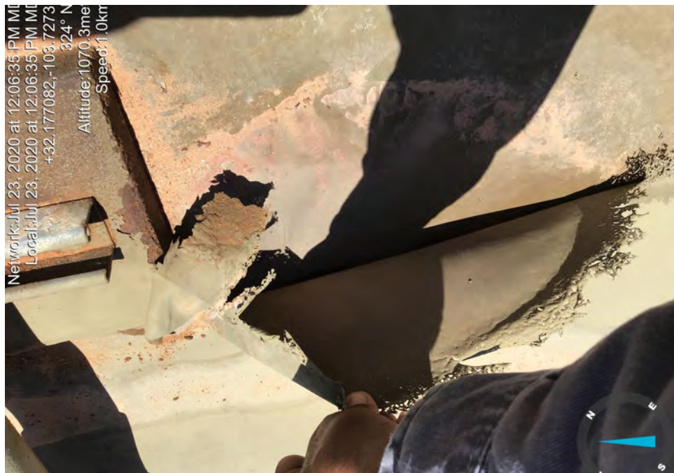
East side, inside pump#3, liner patch unglued
