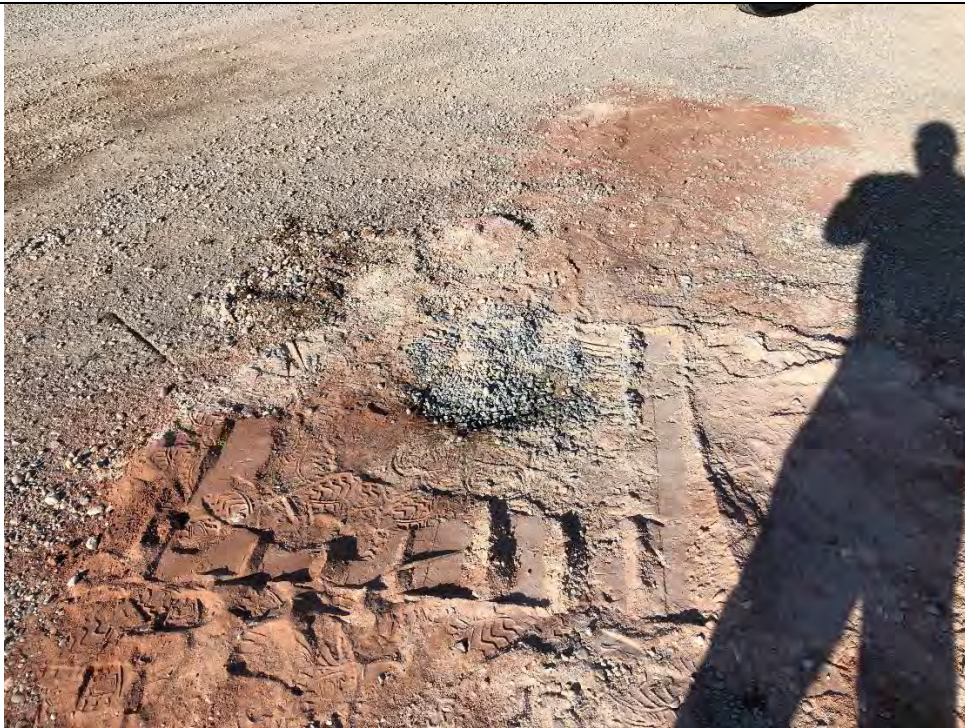
Photo 1: View looking east of SB-East after it was plugged.
