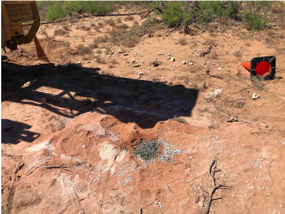
Photo 2: View looking south of SB-South after it was plugged.
